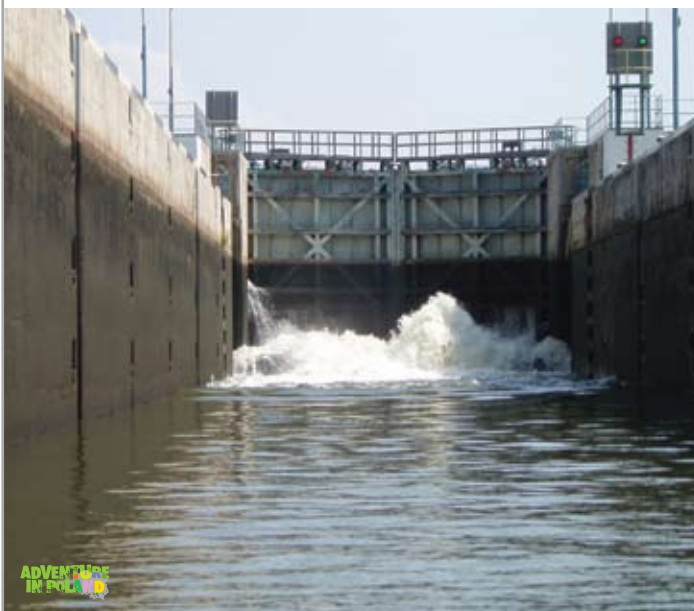
INDUSTRIAL LOCK ON ODRA RIVER
