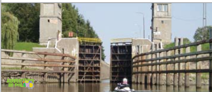
LOCK IN BRZEG DOLNY
